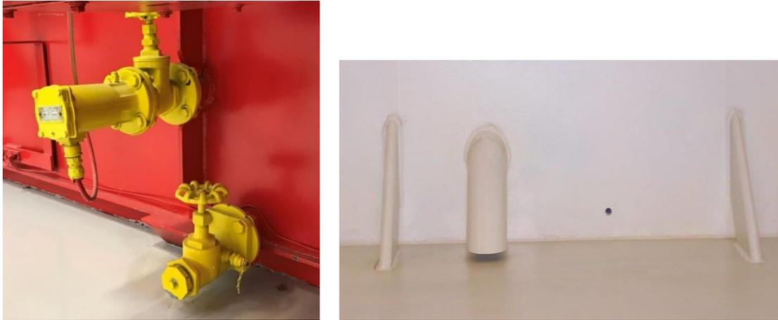
Figure 12 Photos of transformer valves and connected piping inside the transformer tank.
